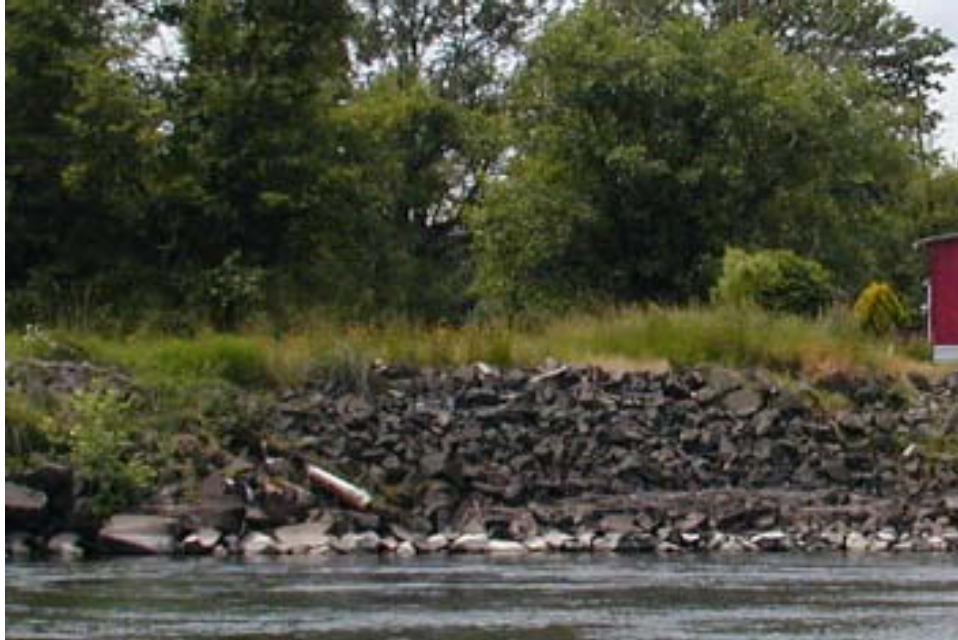
Photo 3. Riparian vegetation and river habitat is modified through actions such as placement of rocks on the bank and removal of trees and other vegetation. (Photo courtesy of Karl Morgenstern, Eugene Water & Electric Board.)
